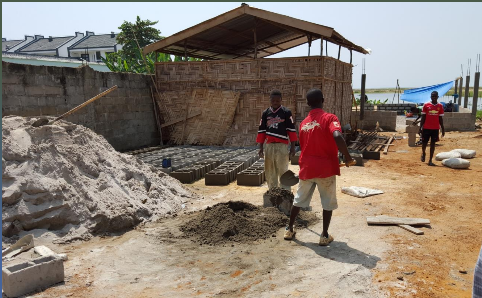
Manually making cinder blocks
