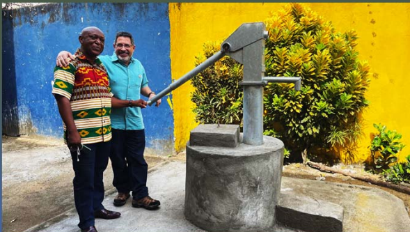
New well with pump at St Paul's
