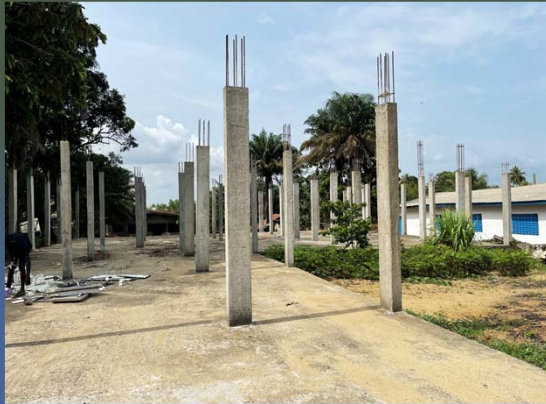
Foundation, with pillars, for the new school!
